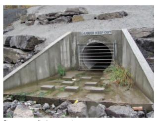
Stormwater discharge outlet
