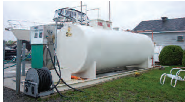
Storage of liquid fuel
