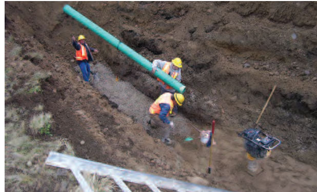
Sanitary sewer pipe installation
