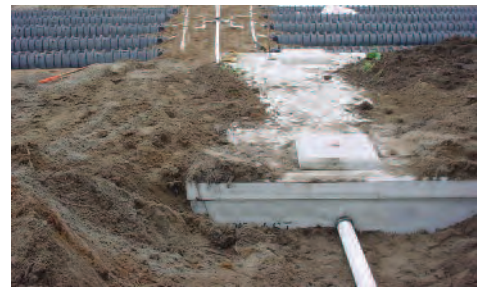
A septic tank and leaching bed
