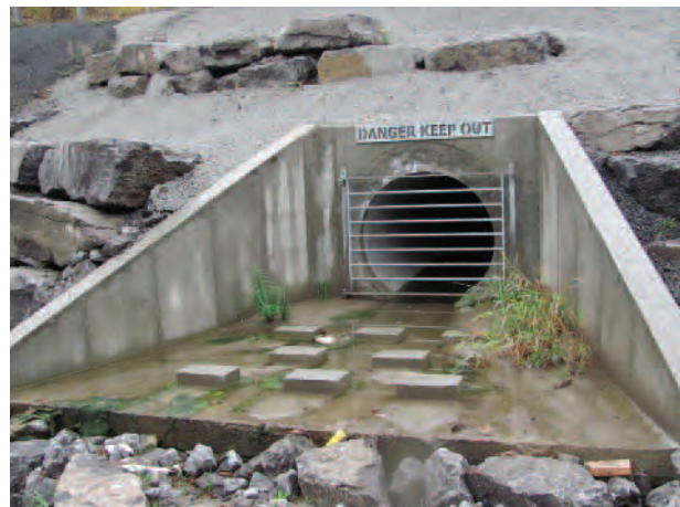
Stormwater discharge outlet
