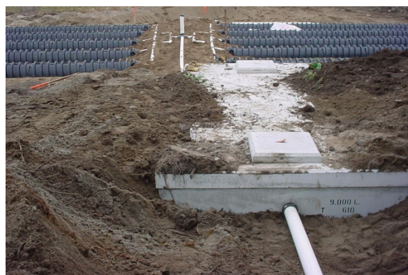
A septic tank and leaching bed
