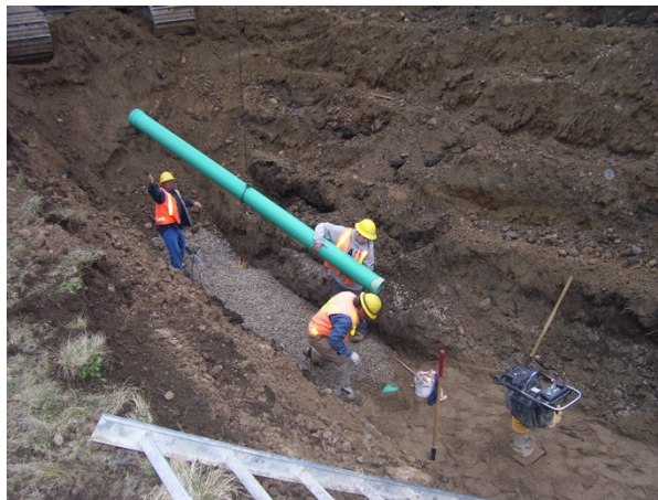
Sanitary sewer pipe installation
