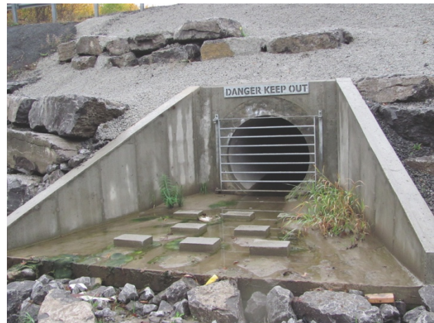
Stormwater discharge outlet
