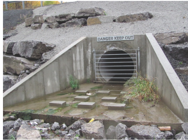
Stormwater discharge outlet
