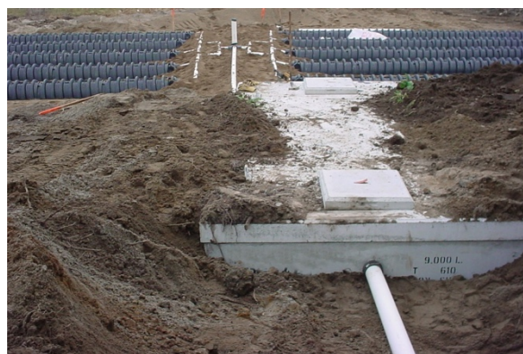
A septic tank and leaching bed
