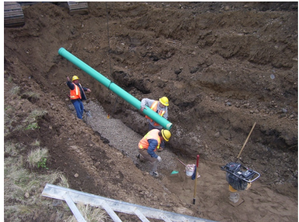
Sanitary sewer pipe installation
