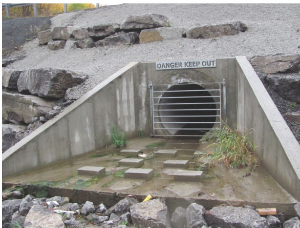
Stormwater discharge outlet
