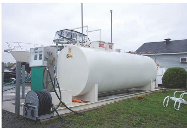
Storage of liquid fuel
