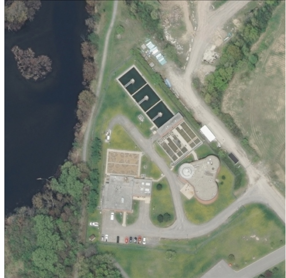
An aerial view of a sewage treatment plant
