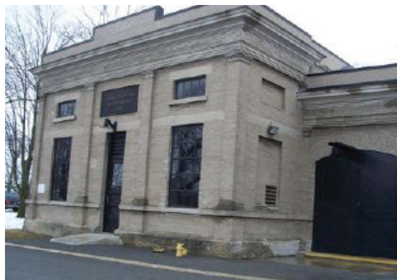
Carleton Place Water Treatment Plant
