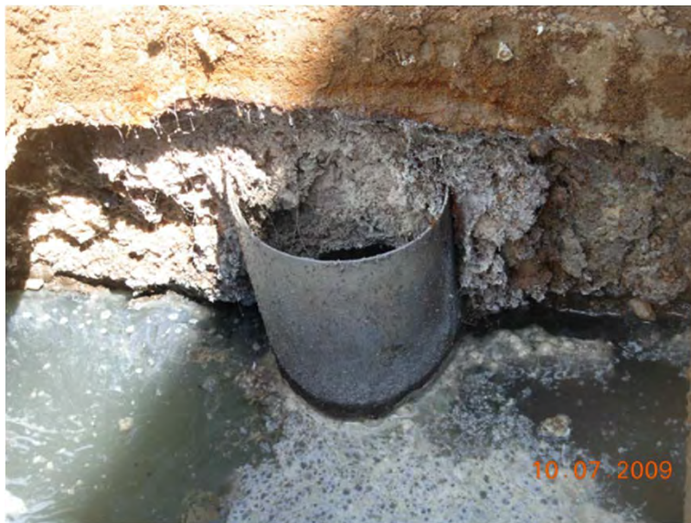
Concrete Corrosion
