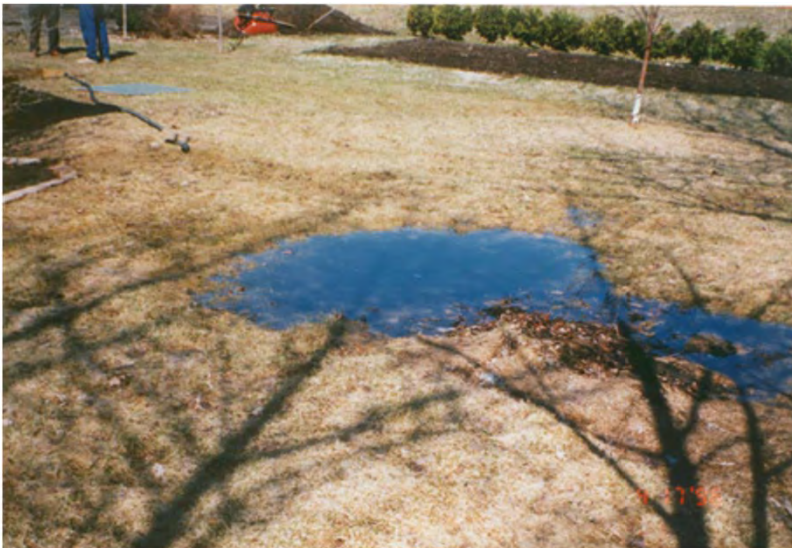
Effluent Pooling Over Bed
