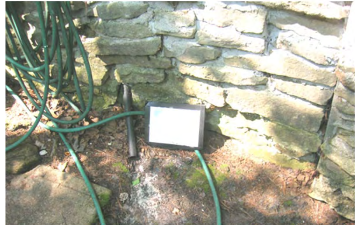
Greywater Discharged to Surface
